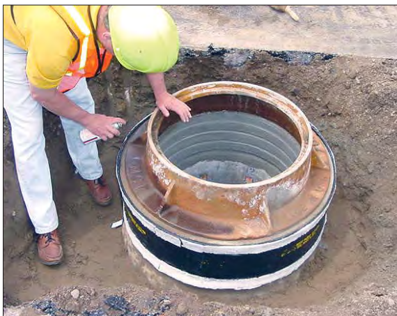
This sequence shows the application of an external rubber manhole seal. From left, the surface is prepared, the seal is pulled into place, and the seal is tapped into final position with a hammer.
