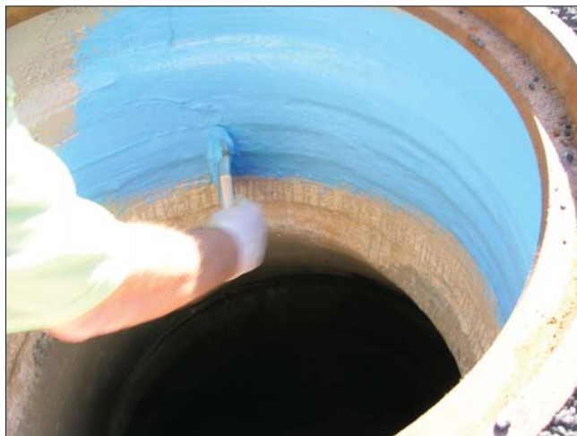
A urethane internal seal is applied to a manhole chimney. The finished project is at the right.
