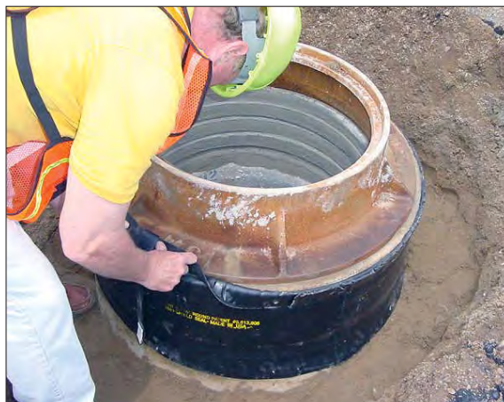
This sequence shows the application of an external rubber manhole seal. From left, the surface is prepared, the seal is pulled into place, and the seal is tapped into final position with a hammer.
