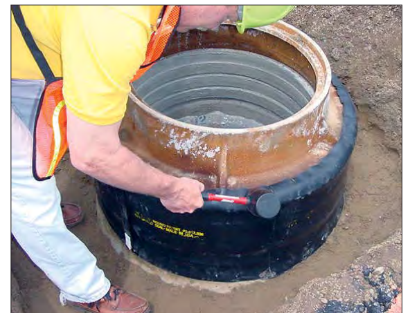
This sequence shows the application of an external rubber manhole seal. From left, the surface is prepared, the seal is pulled into place, and the seal is tapped into final position with a hammer.
