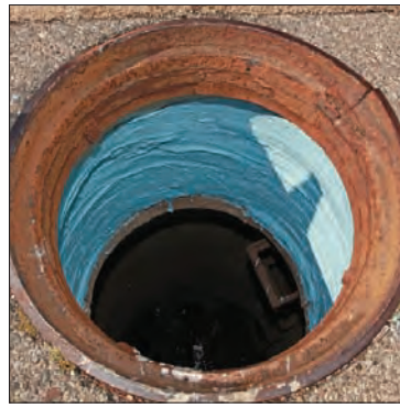
Left, a torch is used to dry the surface before priming of the manhole in preparation for sealing. Right, the manhole surface with the topcoat in place.
